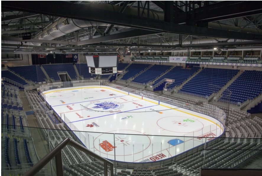
Figure 3: Ephesus LED installation at Ricoh Coliseum in Toronto more than tripled the previous illuminance levels
